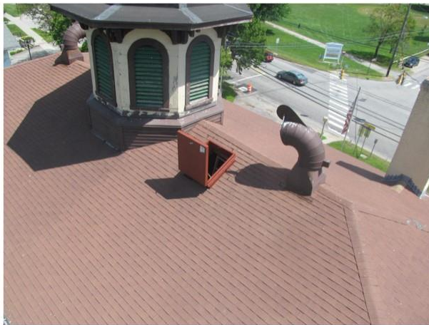
Main roof with new hatch.
