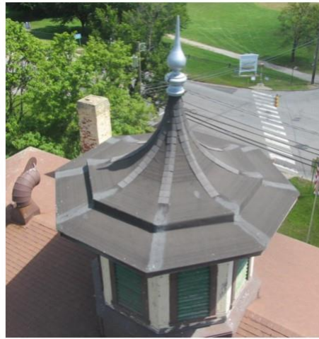
Cupola roof fair condition.
